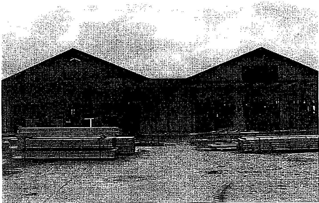
Additional construction underway for the new St. John Elementary School
