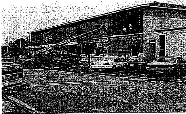
Construction underway at A. M. Barbe High School
