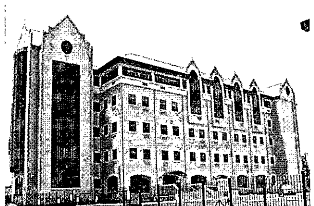
Old Warehouse After Renovations to Create New Residence Hall
