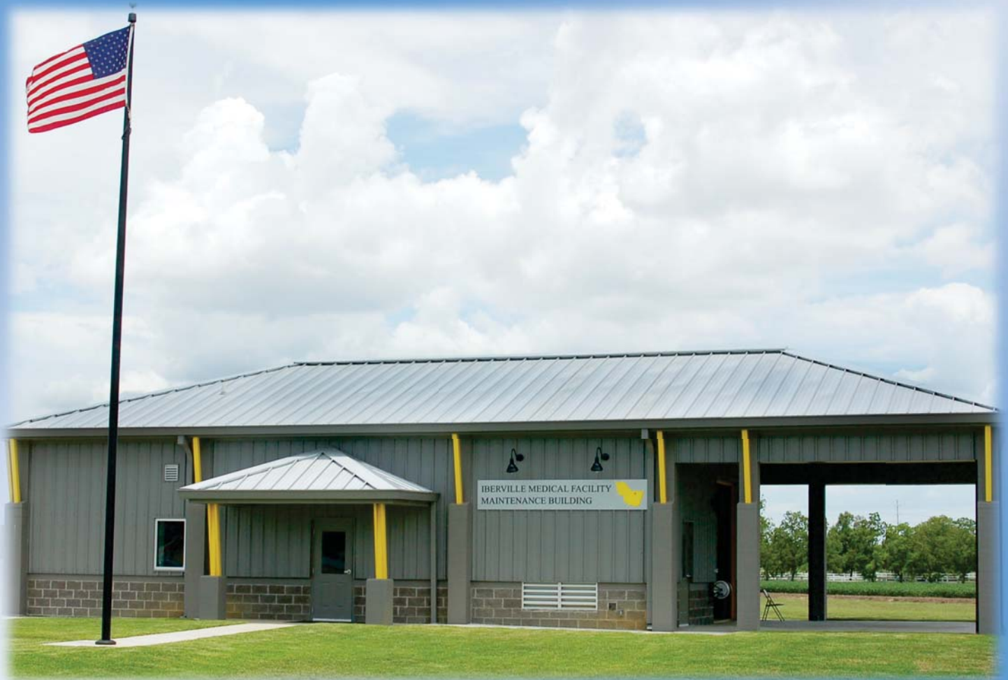
New Maintenance Building—Ochsner Medical Facility
