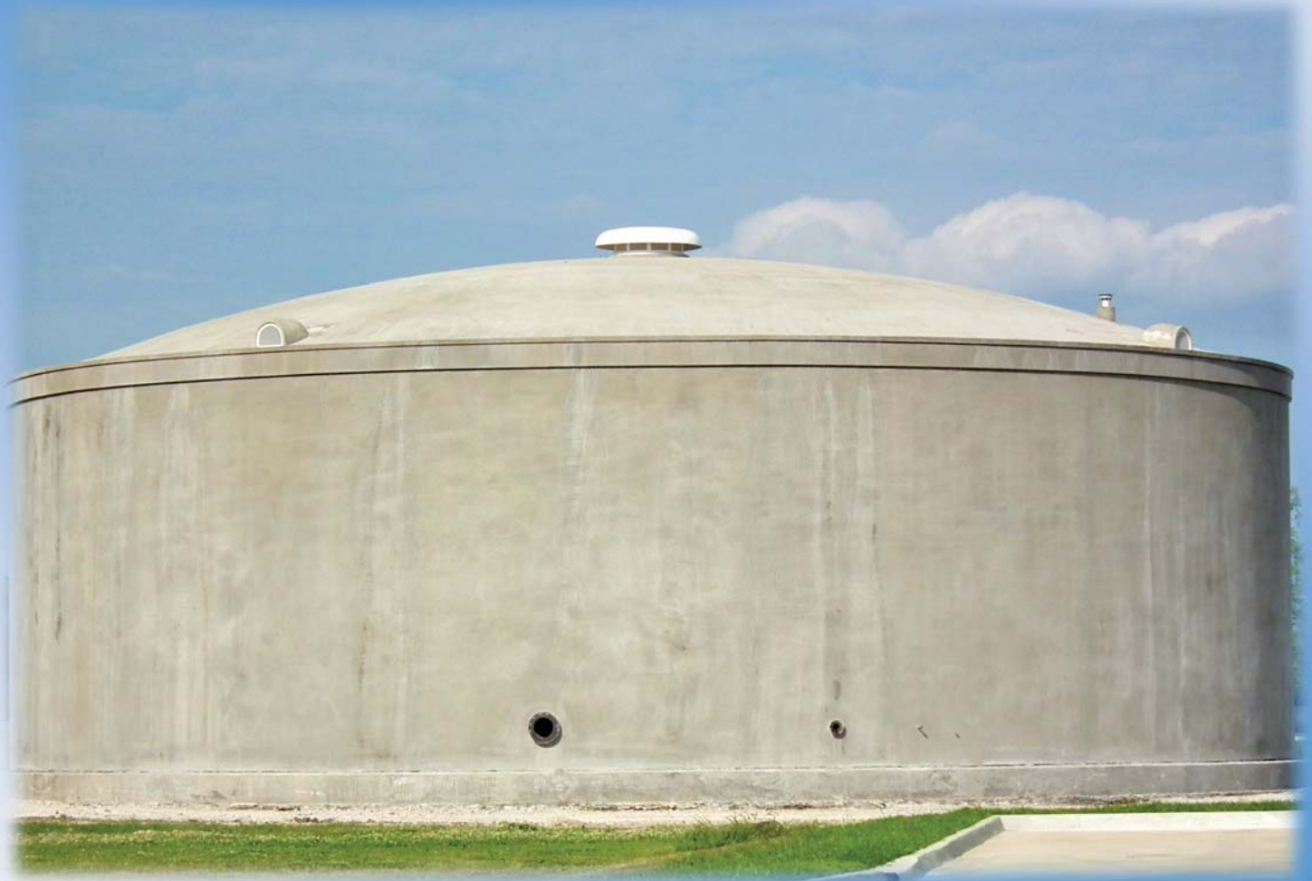
750,000 gallon water storage tank
