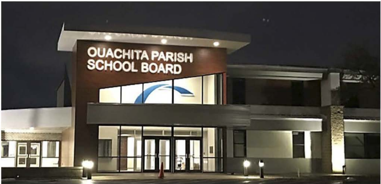
New location of Ouachita Parish School Board Central Office Complex
