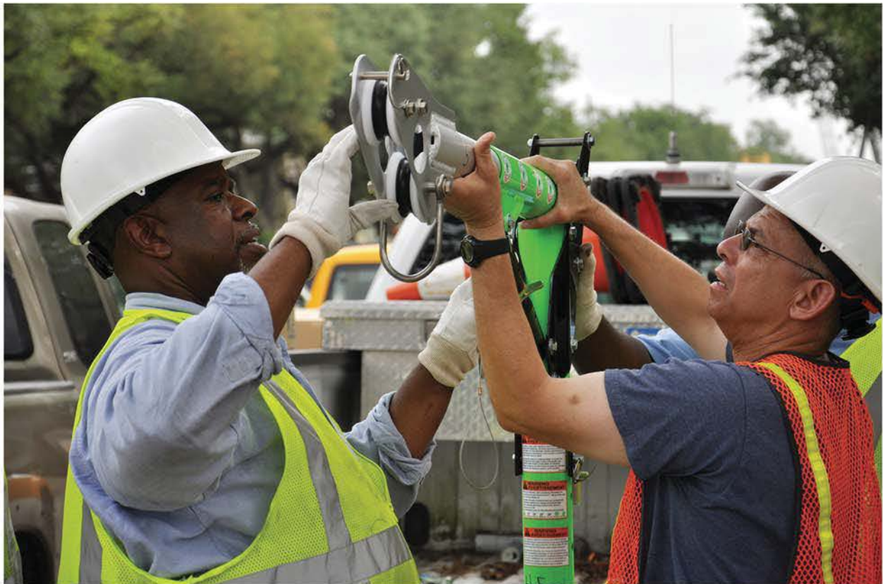
SWBNO safety managers Craig Williams, left, and Joseph Mirabin install a hoist at a job site on Napoleon Avenue in Uptown. Designed for work in manholes and confined space, hoists provide another level of safety for field workers.
